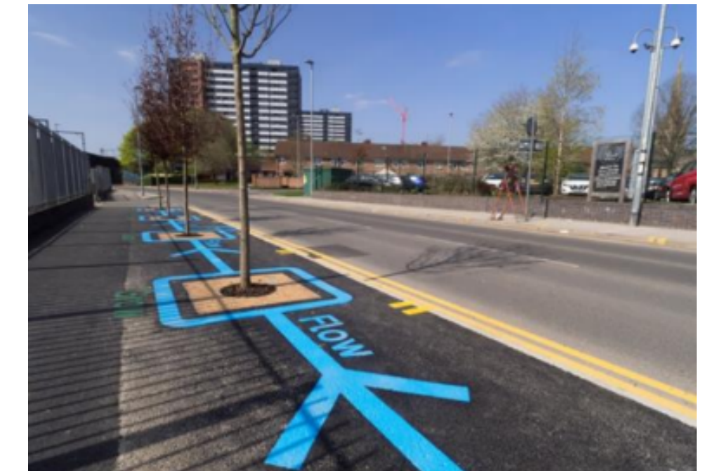
Introducing Sustainable Urban Drainage that mitigates the impacts of climate change and increases biodiversity
