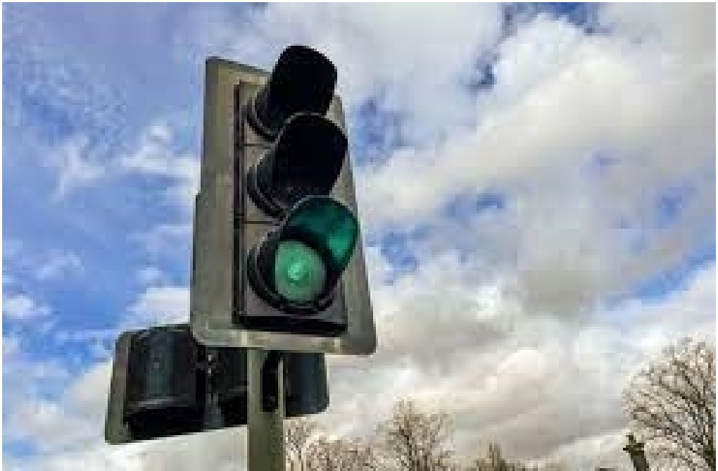
Signal priority for late running bus giving a green wave through signals
