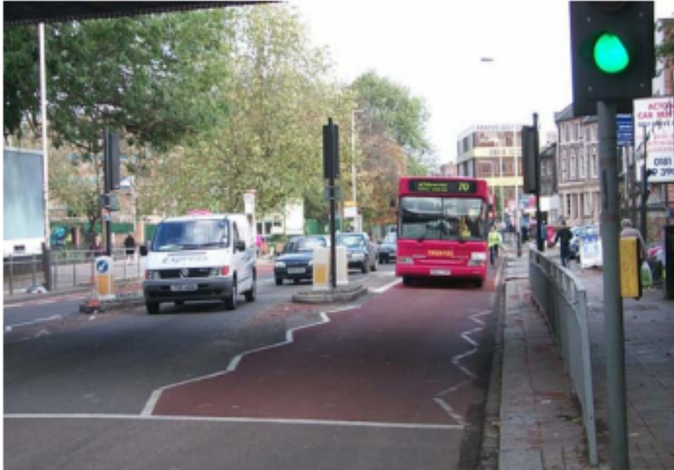
Bus priority at Junctions by moving bus priority to the front of the queue
