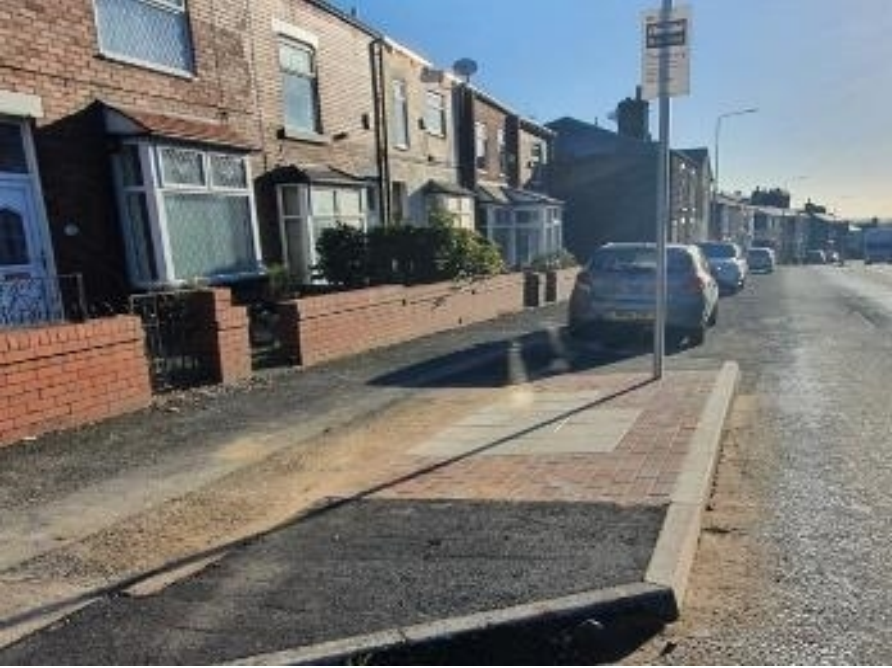
Removing inset bus stops removing the need for buses to merge into traffic
